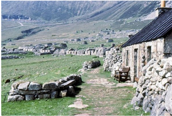
The Village Street showing restoration work
