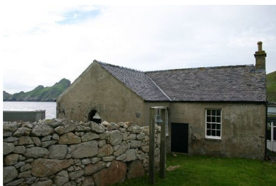
The schoolroom (on the right hand side of the photo) was built as an annexe to the church in 1884.
