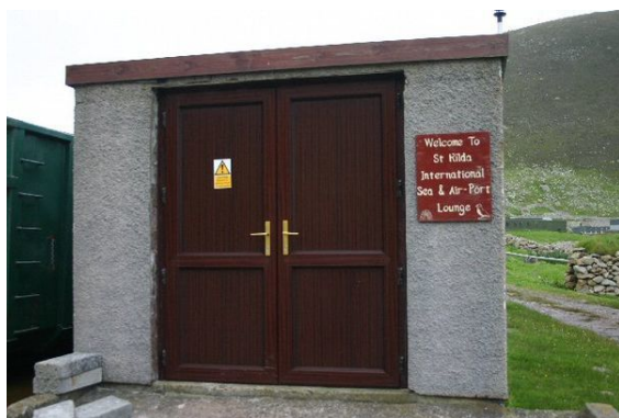
This 'International Sea & Airport Lounge' is situated adjacent to the helipad and landing craft slipway.
