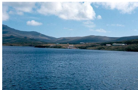
Meteorological station at Beeman Cove (unmanned/automatic since 1995)
